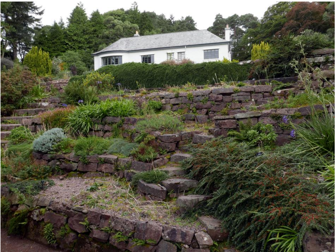
Much of the original rock garden terraces remain intact and it is hoped that in coming years they can be restored.
